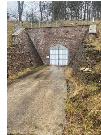
Entrance to drainage tunnel
