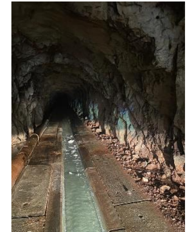
View inside the c. 4x4m drainage tunnel
