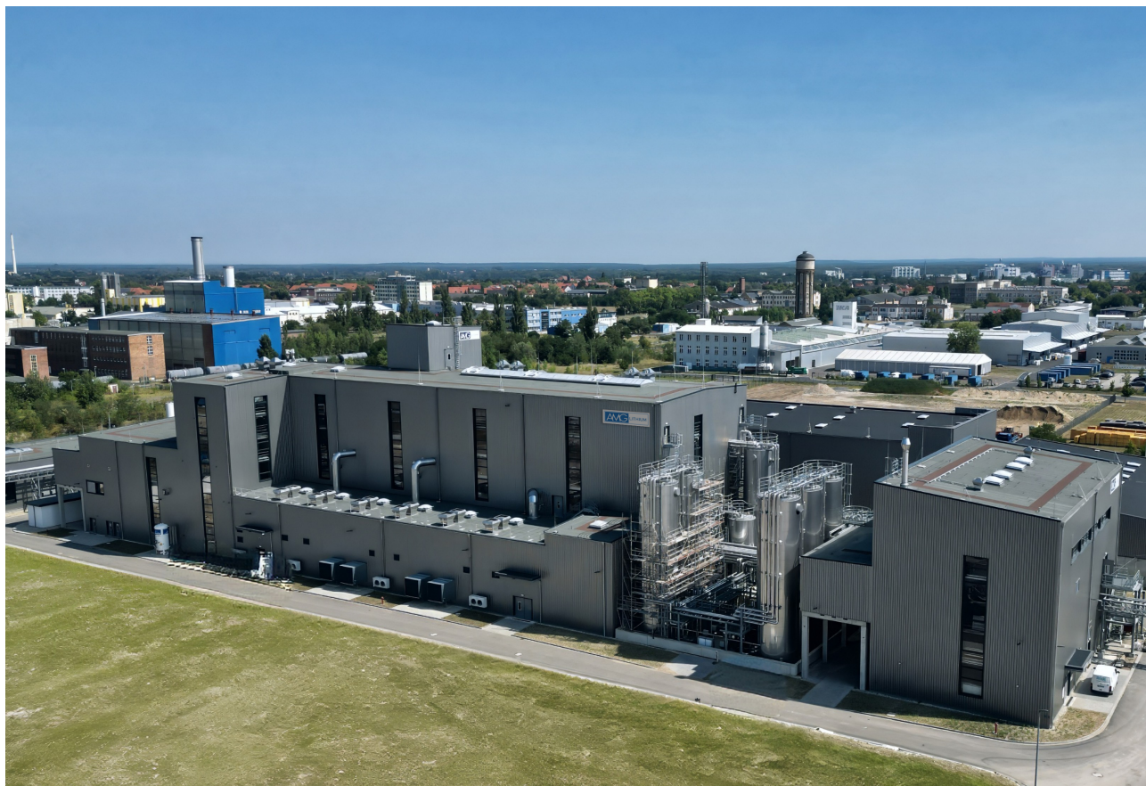
Lithium Hydroxide battery-grade refinery (Bitterfeld, Germany)
